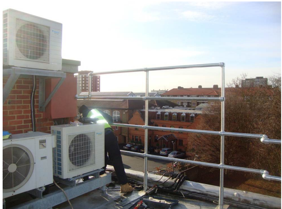
Initial layout and erection of rail to roof edge
